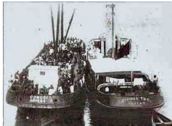
The Tug-boat 'Colonel Thys' transferring workmen at the river estuary
